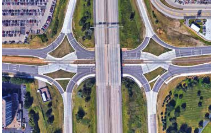
Figure 6: The double crossover diamond (DCD) reduces the number of crossing conflicts from ten to two. Even those conflicts can be eliminated with small overpasses. This aerial photo shows the 34th Avenue and I-494 intersection in Bloomington with crossovers bisected by light-rail tracks. Source: Google maps.
