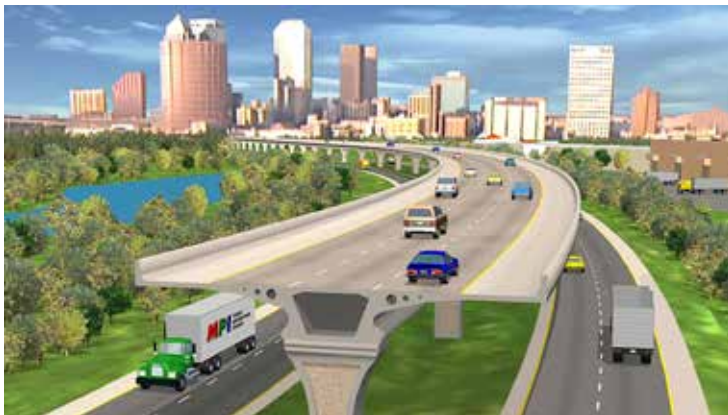
Figure 5: Elevated freeway lanes built in the median strip of an existing freeway, thus saving the cost of purchasing additional right of way. This example shows three reversible lanes serving inbound traffic in the morning and outbound traffic in the afternoon. If traffic is more balanced, the elevated structure is wide enough to allow for four lanes, two in each direction. Source: Tampa-Hillsborough Expressway Authority.
